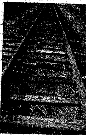
A VIEW up the tracks near Brownfield.
